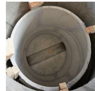
4. Next, glue the two smaller, straight parts on all sides to the polymer concrete elements that have already been placed.
