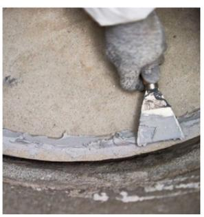
All joints between the ring segments shall be connected with DURA.Glue to ensure a watertight and robust system. Before applying the DURA.Glue, care must be taken that the area where the glue will be applied is dust-free.
