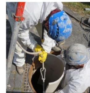
The necessary safety measures must be observed during insertion of the elements into the manhole. It is recommended to use a small crane to lift all panels inside.
