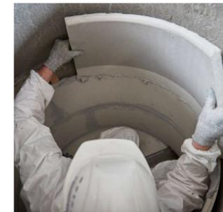
1. First mark the center of the slope and the straight line of the existing cone part before you put on the new cone.
